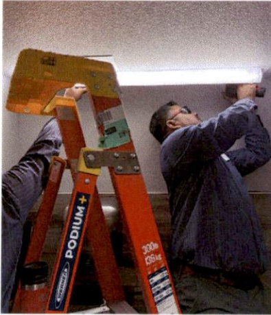
Installation of a light at the bathroom at the Senior Center.
