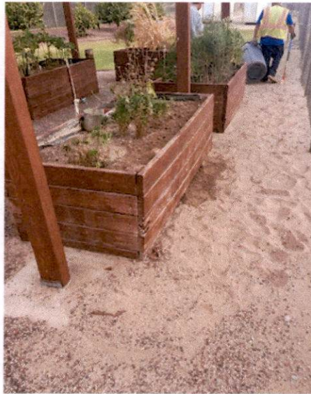
Assisted the Senior Center in repairing a wooden planter
