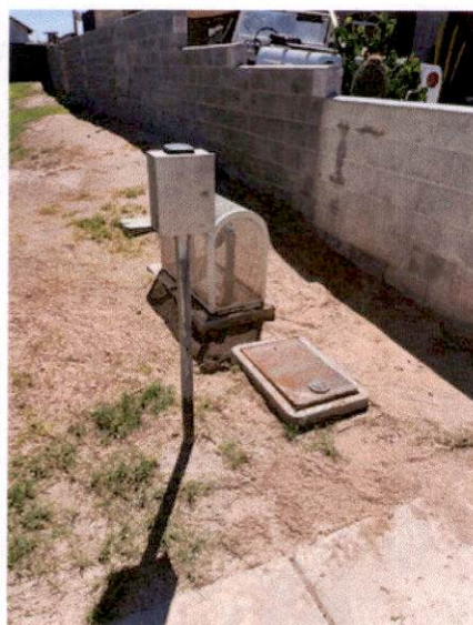
Water leaks were repaired at several backflows
